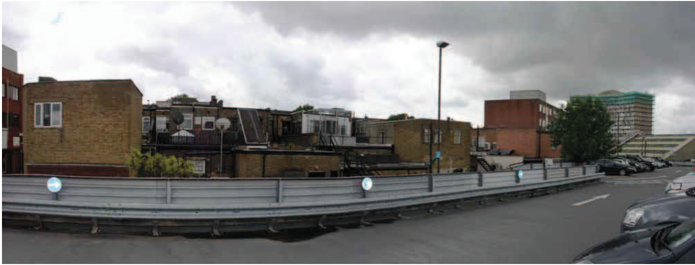
Figure 2: Rear of 46-64 London Road viewed from Peel House Car Park
