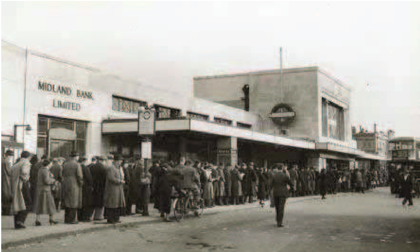
Figure 9: Morden Station, 1934, with addition of bus canopy. (London Transport Museum)
